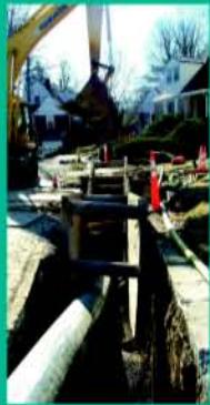
Neighborhood Construction Projects
