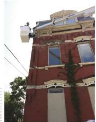
Deconstructing exterior from the facade of 1777 Queen City Ave.
