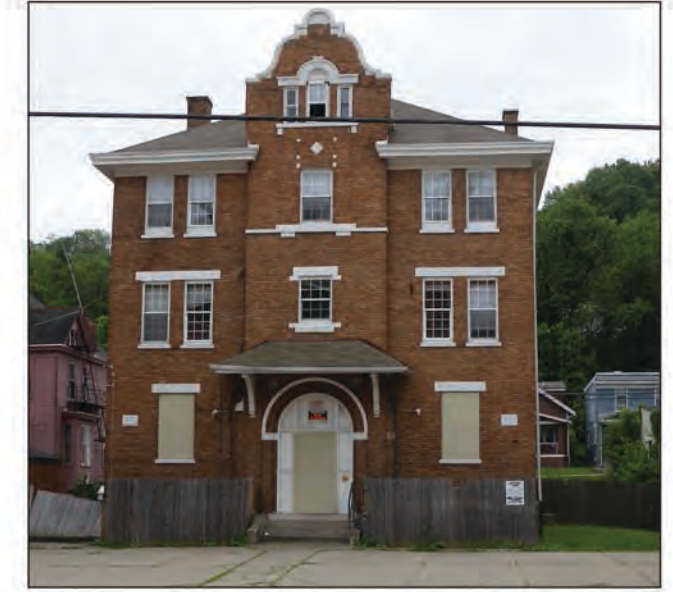
1789 Queen City Avenue (nun's house)
