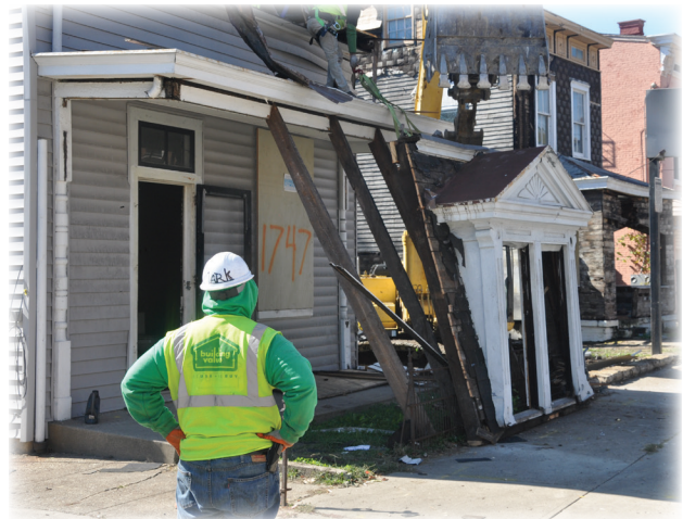
Deconstruction of a building in South Fairmount
