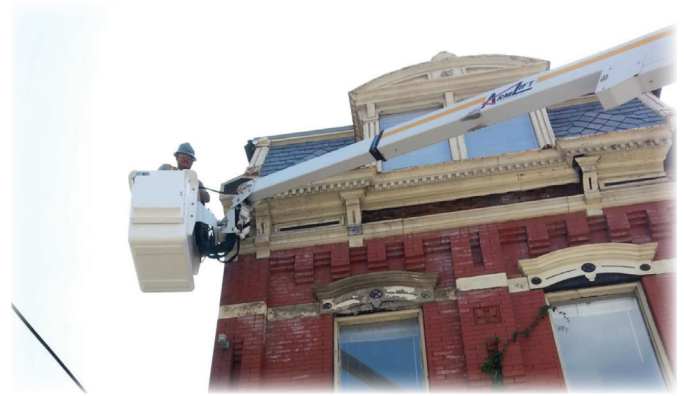
Soft stripping the exterior of a building in South Fairmount
