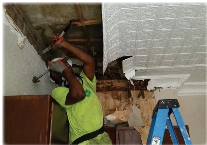
Trainees softstripping buildings for reusable materials
