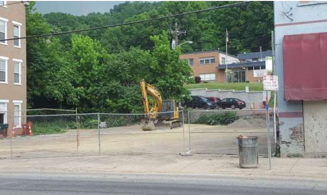
Completed Deconstruction of 1608 Queen City Avenue
