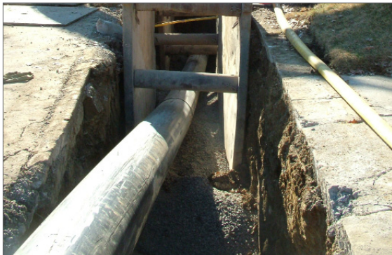
Photo depicting "open cut" method of construction.
