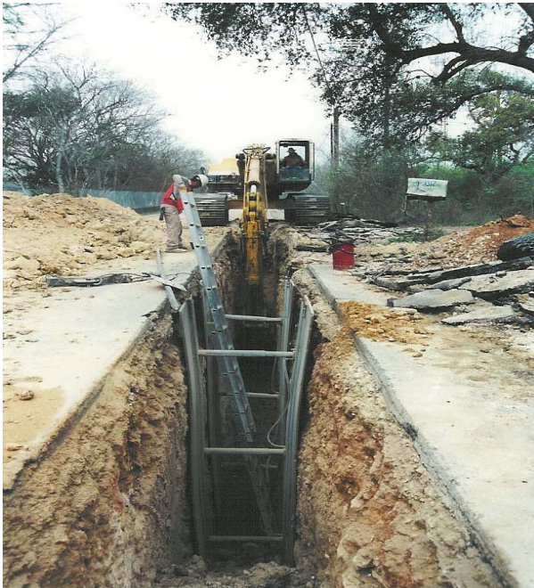
Trench Method within public right of way
