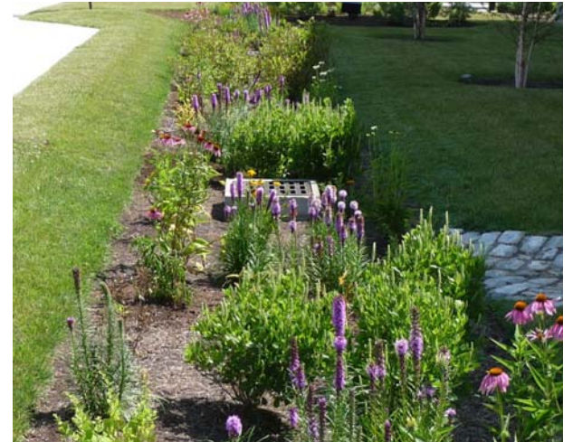
Rain Garden Inlet
