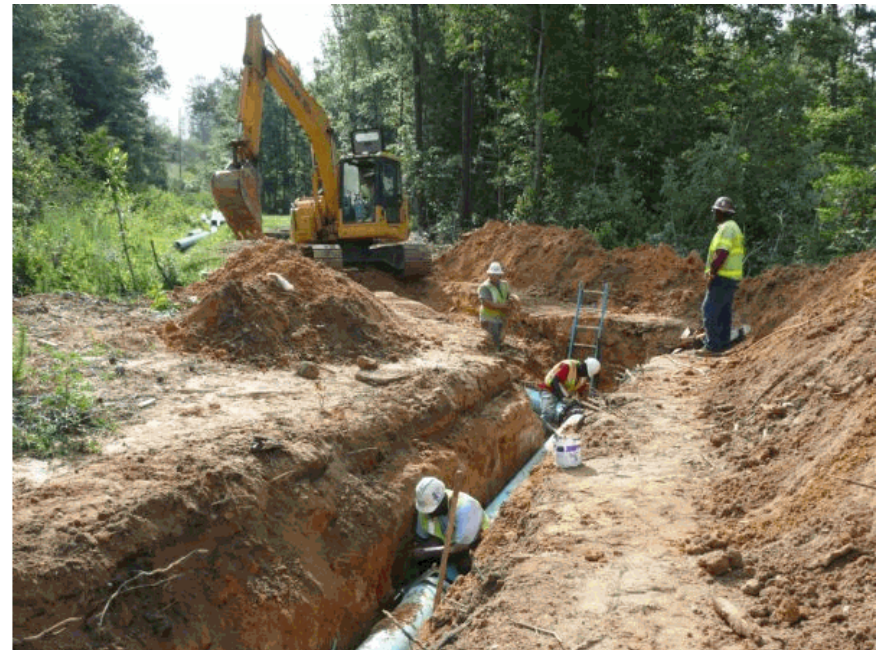
Trench Method outside of public right of way
